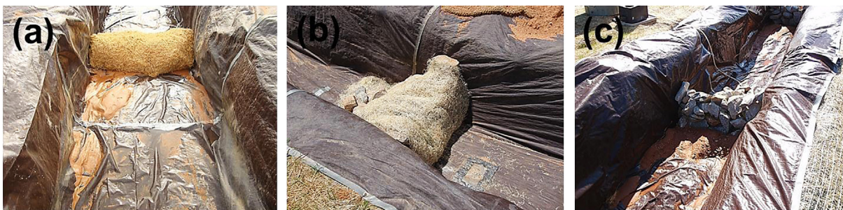
Fig. 2. Check dam types tested: (a) excelsior wattle, (b) rock check dam wrapped with excelsior erosion control blanket (ECB), and (c) rock check dam.
