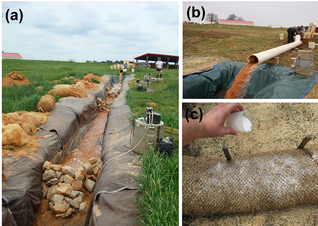
Fig. 1. Experimental setup showing (a) a drainage ditch installed with rock check dams, (b) turbid water generation by adding sediments, and (c) application of polyacrylamide on an excelsior wattle.
