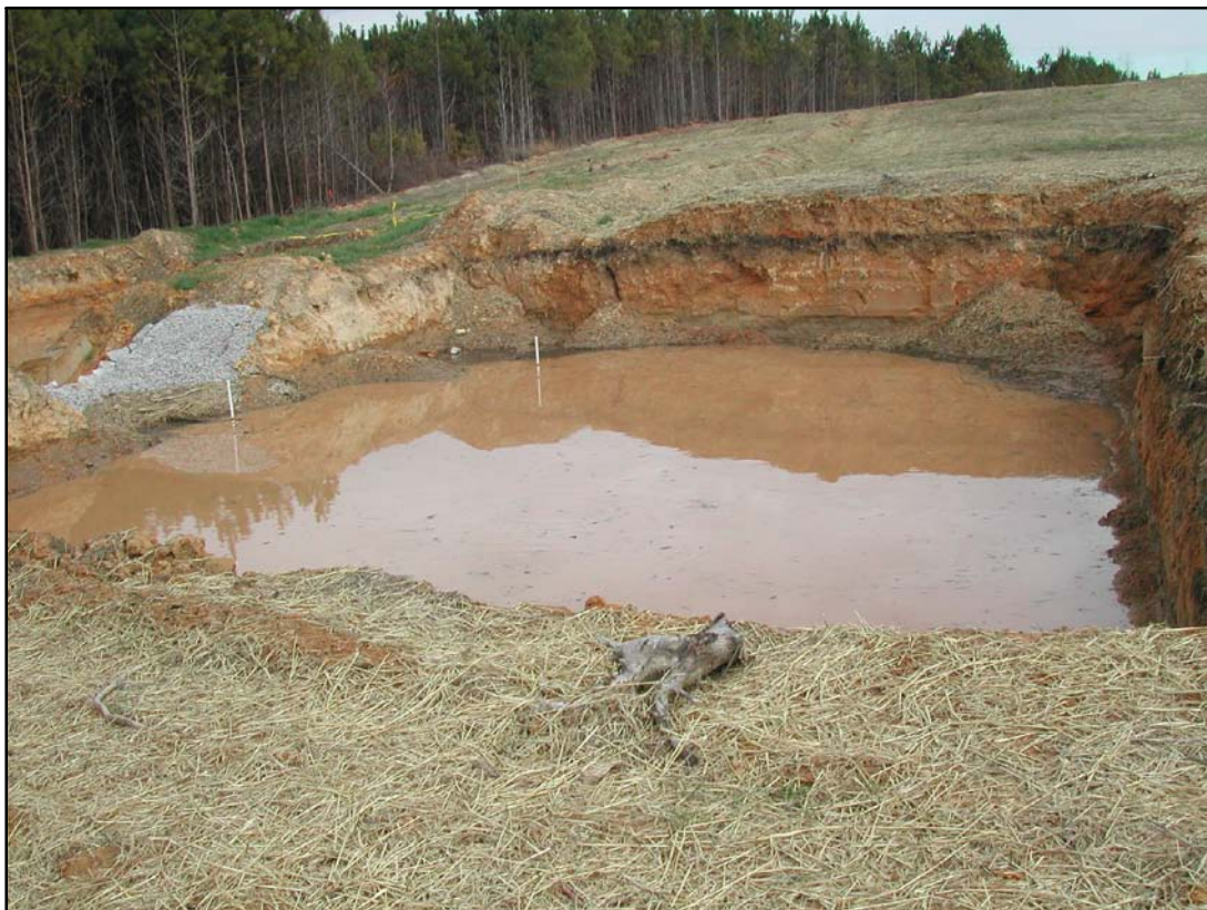
Figure 2. Standard 10-year trap (10ST) on 12 December 2005, when the water was less than 0.3 m deep.
