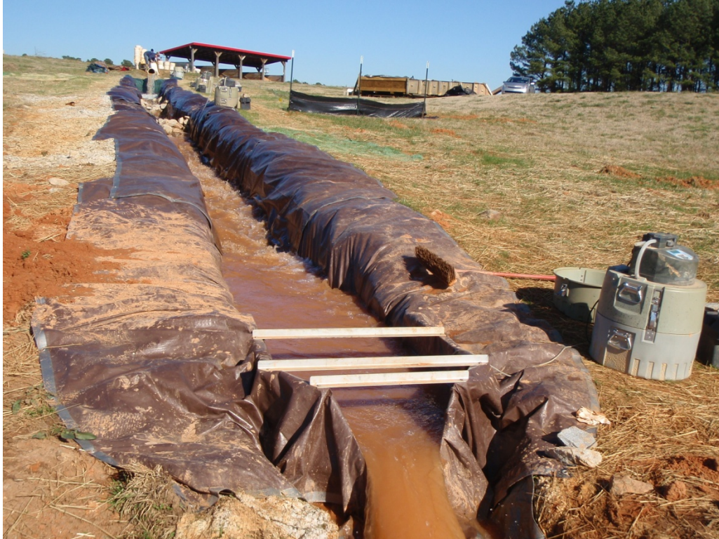
Figure 1. Example of rock check dam test at peak flow.
